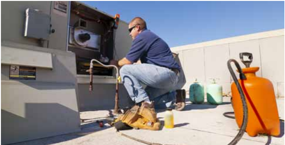
Figure 7: Servicing a rooftop system
