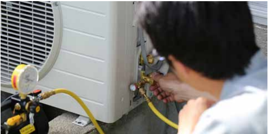
Figure 6: Changing refrigerant in air-conditioning unit
