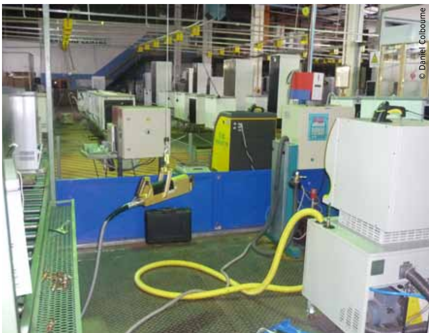
Figure 4: Charging equipment on a production line
