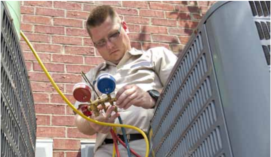
Figure 5: Charging HCFC-22 into an air-conditioning system
